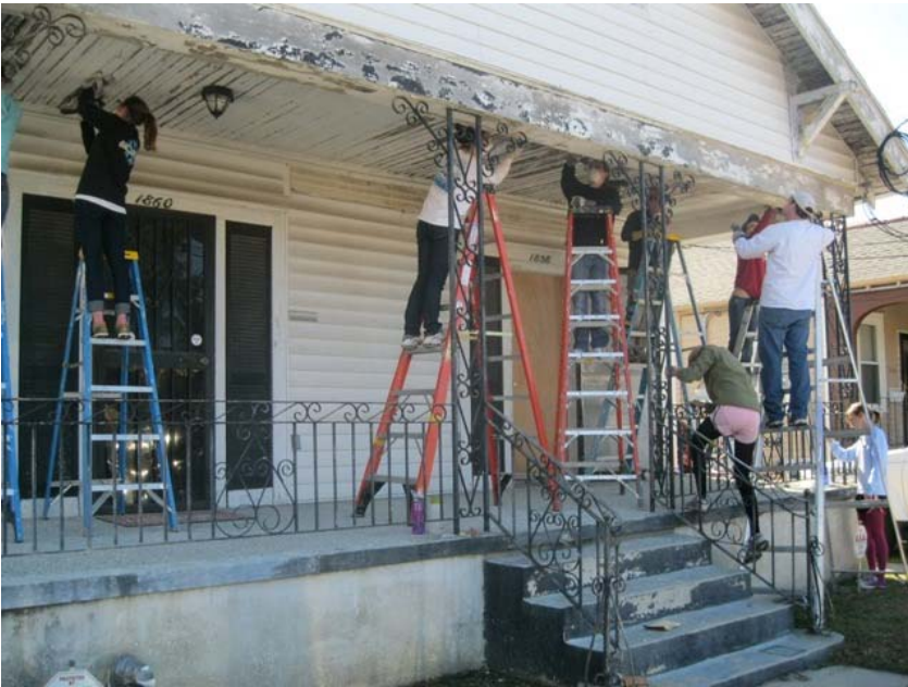
Scraping and sanding
