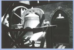
The bell is made of copper and tin, weighs 1500 pounds, and has a diameter of  $40 \frac{1}{2}$  inches. It rings on the note of "G".
