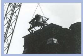
When the bell arrived at the church, it became apparent that it would be impossible to take it up the narrow stairway of the bell tower. Consequently, a hole was cut in the roof of the bell tower and the bell was raised by a crane and lowered into place.
